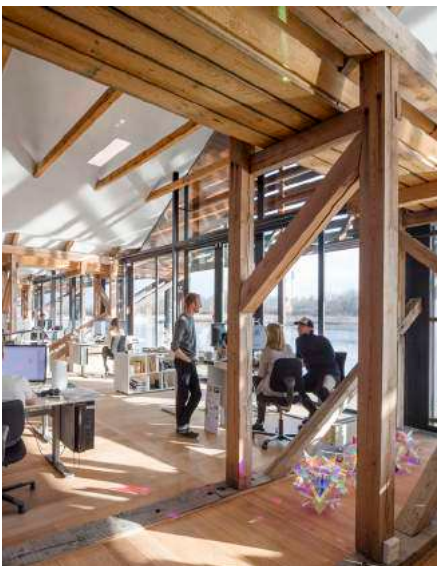
Photos: The connections in the timber structure are made as traditional joints with bolts and carvings that easily can be disassembled.
