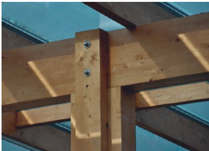
Photo: Visible connections designed for disassembly is part of the architecture.
