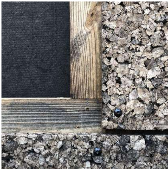
Photo (right): Facade build up using MDfacade expanded insulation cork panels mounted on timber battens.
