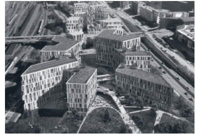
De Fire Styrelser 3XN Architects, Kalvebod Brygge, Denmark 2014, Offices, 42,000 m 2
