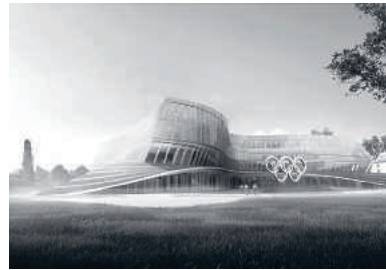
IOC Headquarters 3XN Architects, Lausanne, Switzerland 2014 Offices, 15,000 m 2
