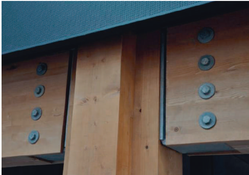
Photo: Visible connections designed for disassembly is part of the architecture.
